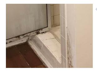
The walls outside my shower are damp and spongy, drywall is bubbling, or damaged. There is evidence of moisture damage and mold/mildew on the wall(s) on the other side of the shower.
